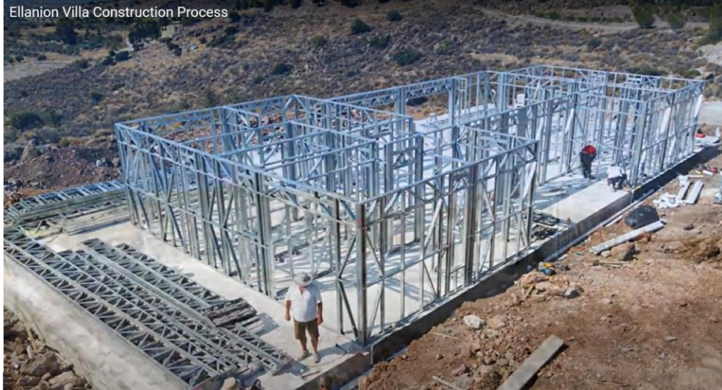
Ellanion Villa Construction Process
