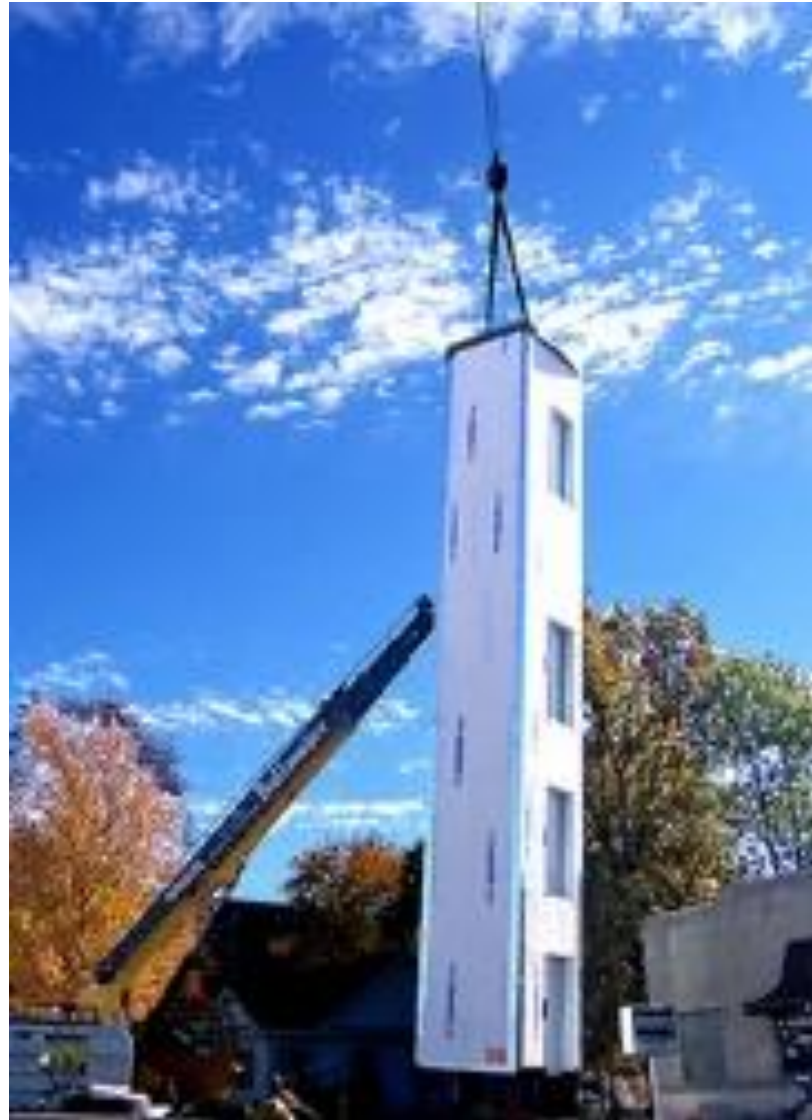
■ New lift added to an old building
