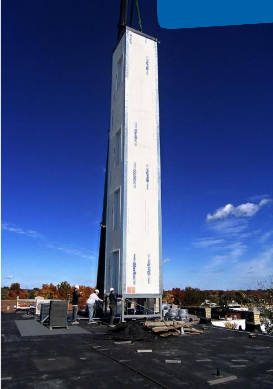
■ New lift added to an old building
